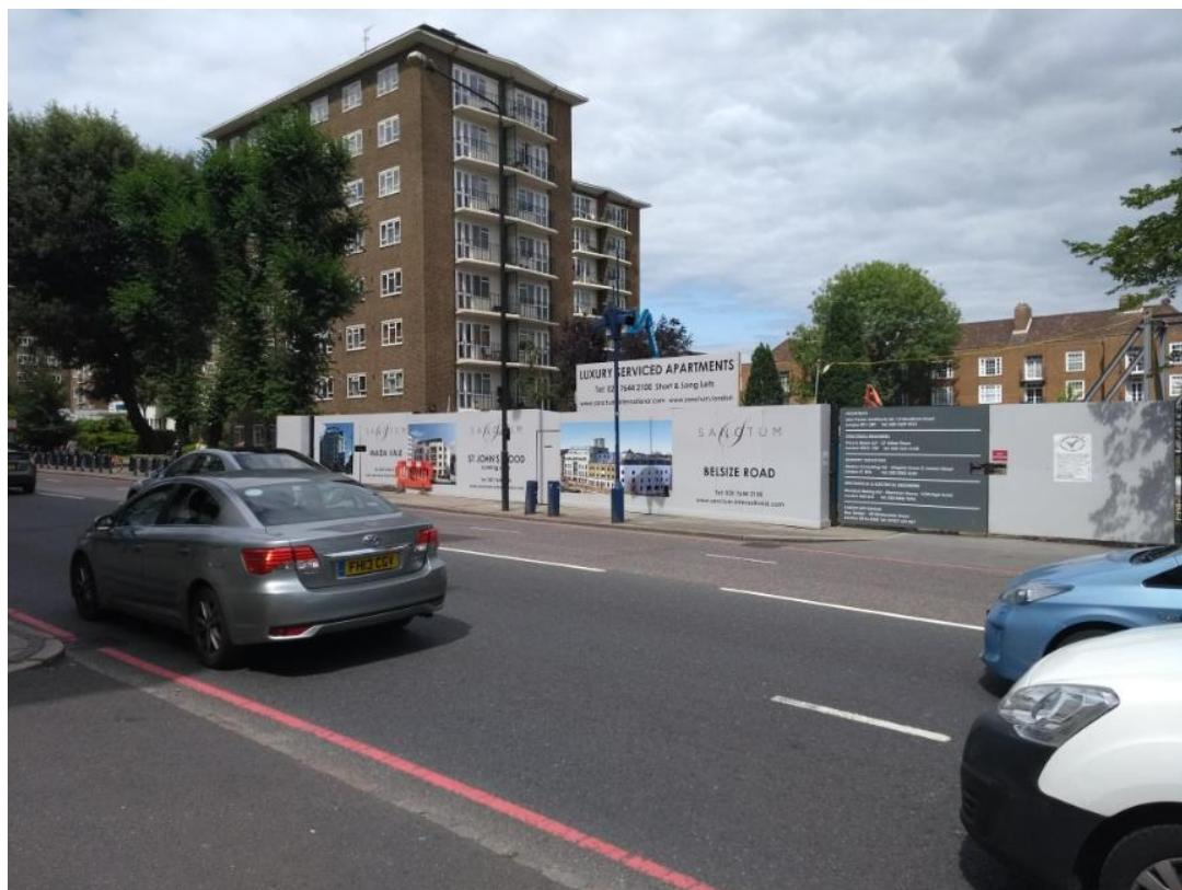
View of site from Wellington Road following demolition of the previous building pursuant to the February 2017 permission.
