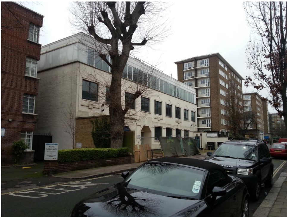
Prior to demolition views of the site from Wellington Road (top) and Cochrane Street(bottom).
